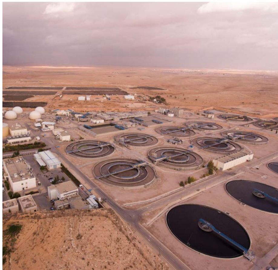
The As-Samra wastewater treatment plant, Jordan.
